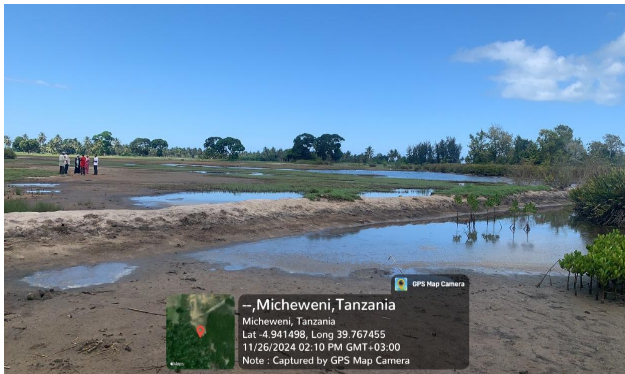
PLATE 2: SAND EMBANKMENT CONSTRUCTED BY SHEHIA TO PROTECT RICE FARMS FROM SEAWATER INTRUSION
