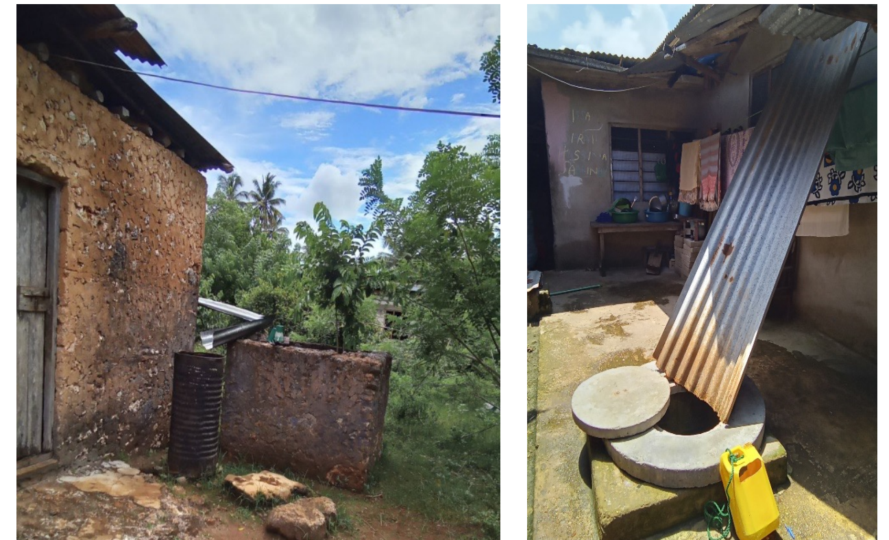
PLATE 1. TRADITIONAL ROOFTOP RWH USING MIKINGO AND MAHODHI
